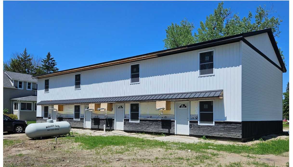
Henderson Apartments exterior — nearing completion
