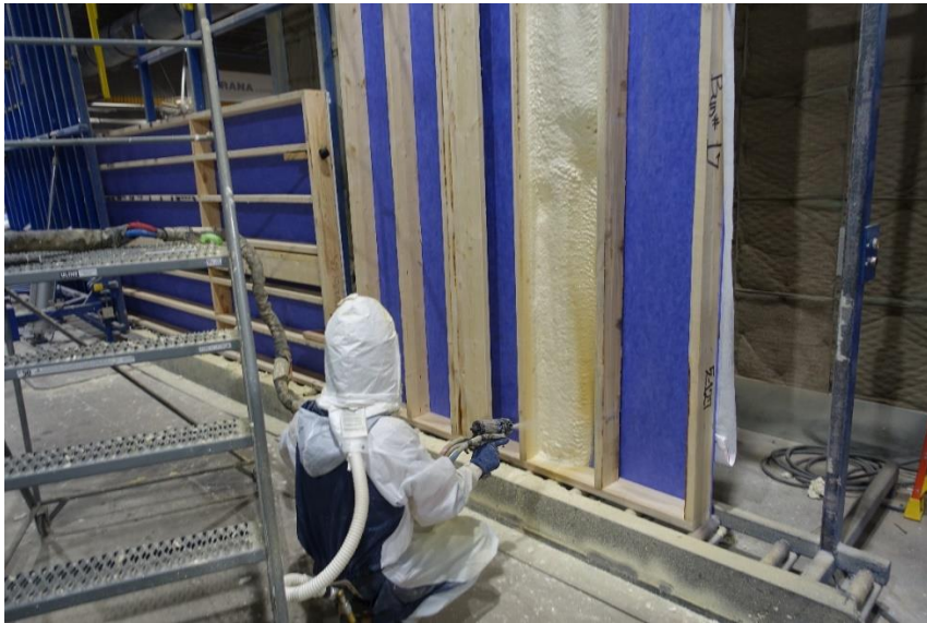
Spray foam application at the factory
