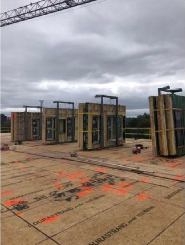
Wall panels in transport frames on the second deck at Hillside
