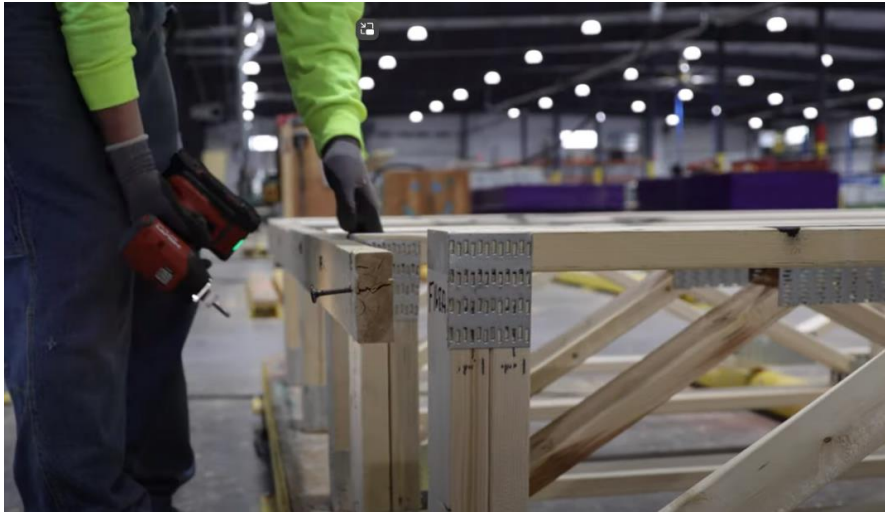
Assembly of a floor section.
