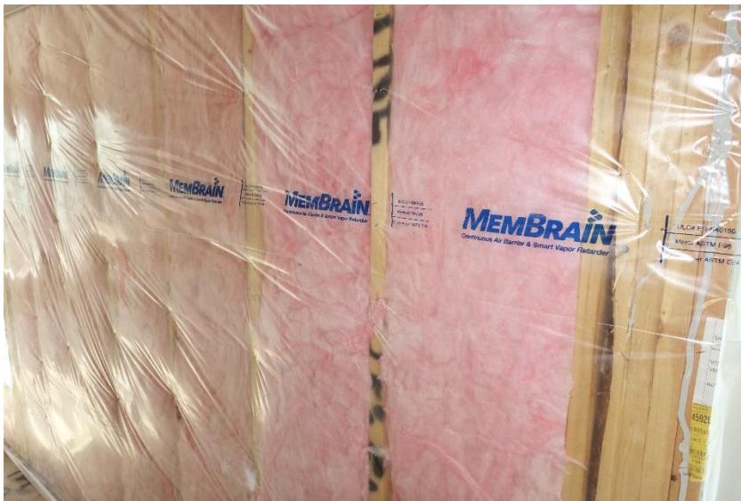
One-hour exterior wall at Hillside Heights
