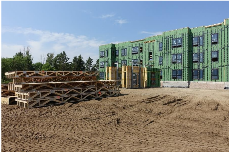
Wall panels stored vertically in racks; floor sections stacked awaiting installation.
