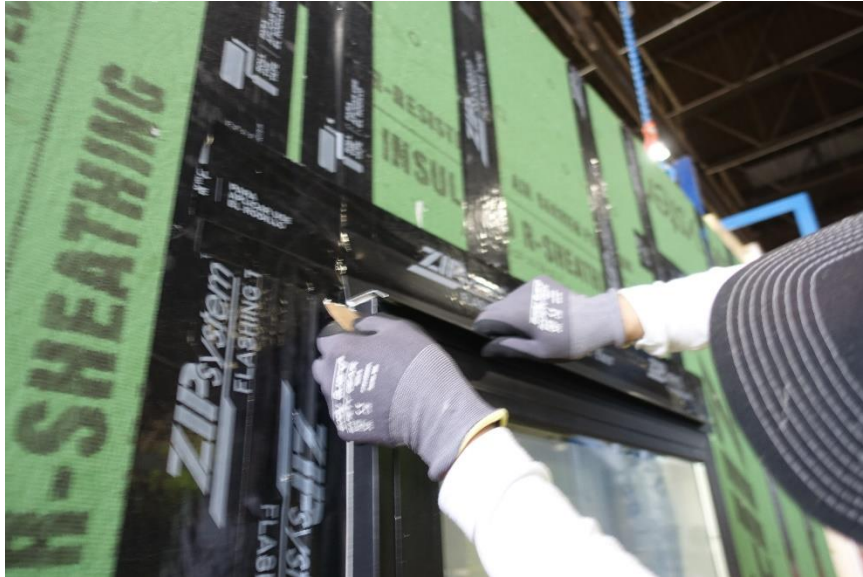
Wall panel with sheathing attached and joints and nail heads tapped.
