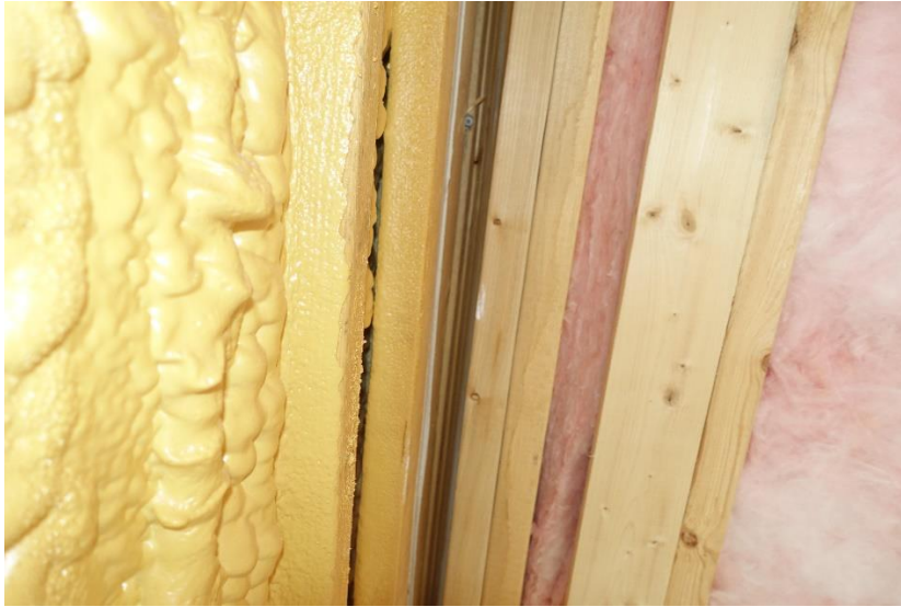
Typical panel to panel joint looking from the interior.
