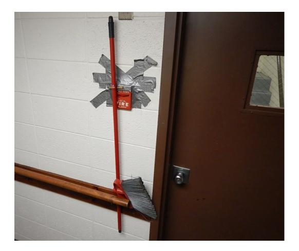
"Example of a patchwork fix actually orchestrated by the fire marshal himself to keep the building operational when a resident pulled the fire alarm and the whole device came out of the wall."
